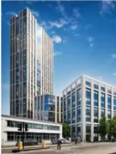
140 Wates Farm Road (Imperial Site)
