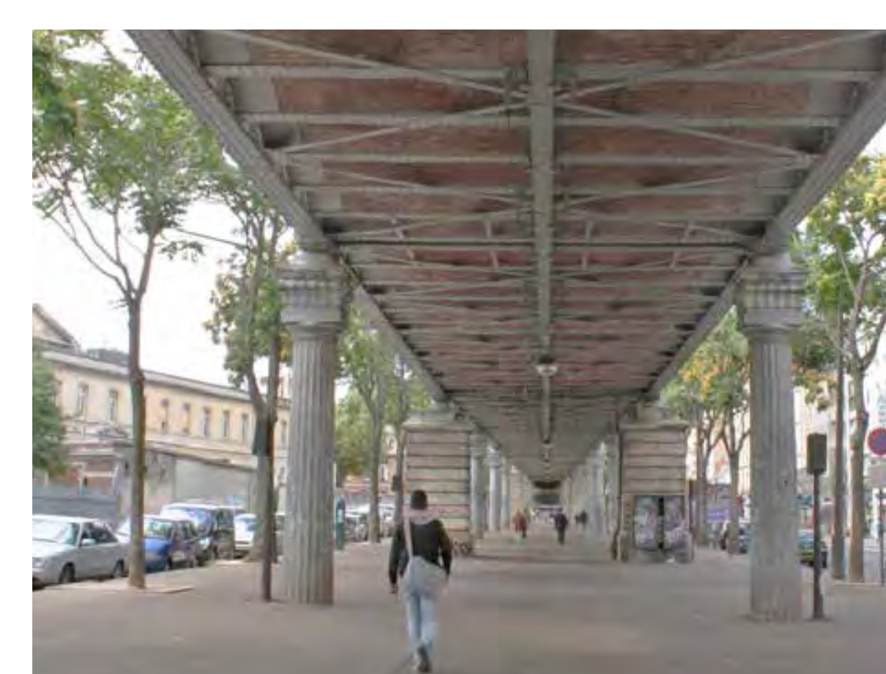
Example of viaduct structure at Boulevard de La Chapelle, Paris
