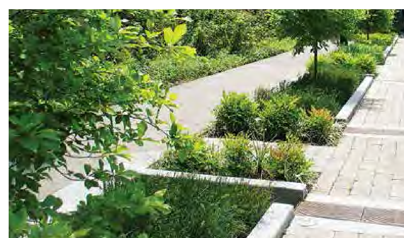
Example of SUDs integrated within the urban environment
