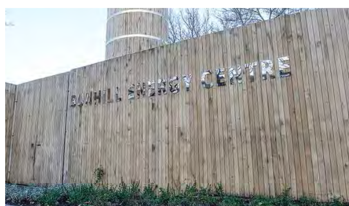
Bunhill Energy Centre, London
