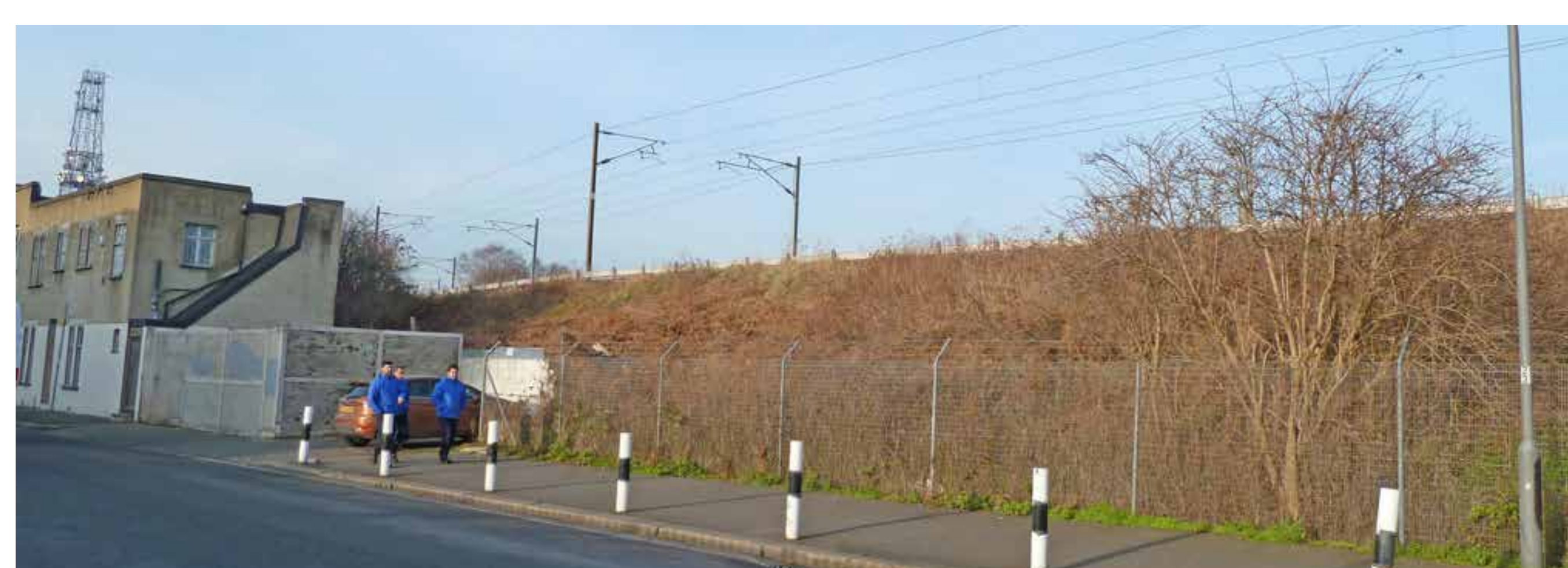
Existing railway embankment
